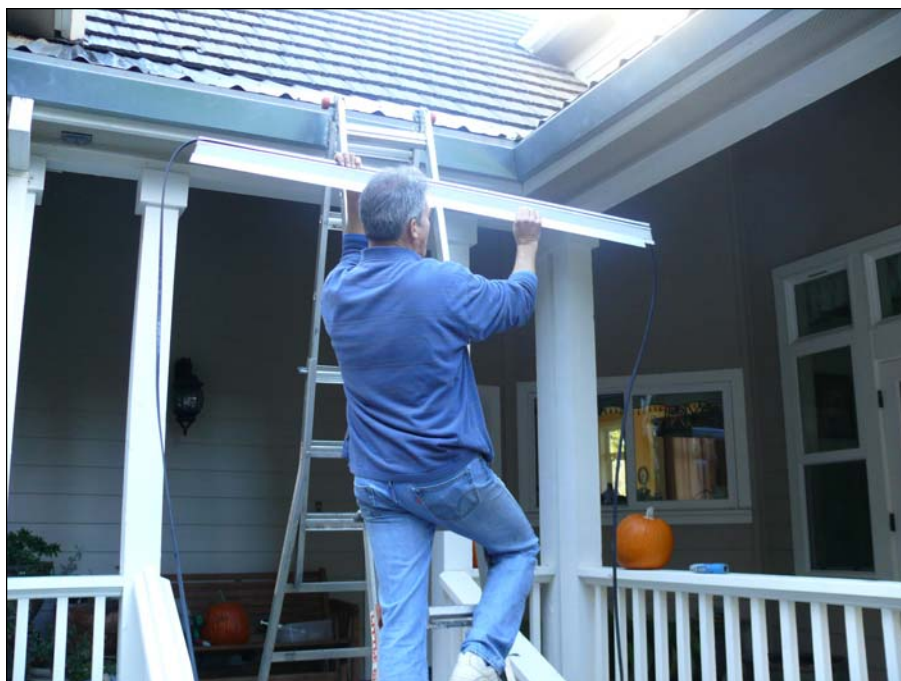
Gutterglove IceBreaker “Walkway” version with the larger mesh size is to be installed over all walkways where pedestrians may walk.
